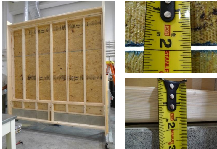
Figure 7. Inner side of baseline wall (left), \sim 1/8'' -wide horizontal OSB joint (top right), and \sim 1/8'' -wide joint between mud plate and CMU (bottom right).
