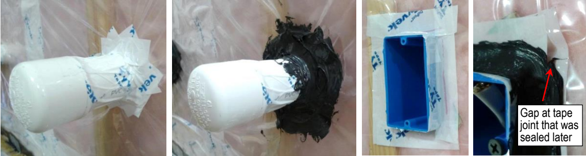
Figure 16. Penetrations through membrane sealed with tape and sealant.
