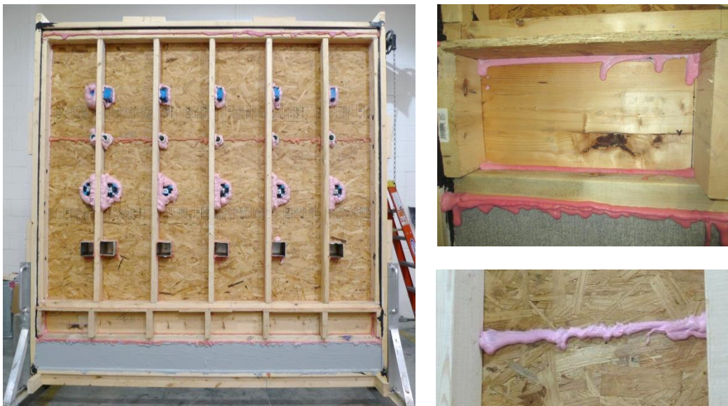
Figure 21. Test wall with OSB as the air barrier material and latex foam sealant at OSB joints.
