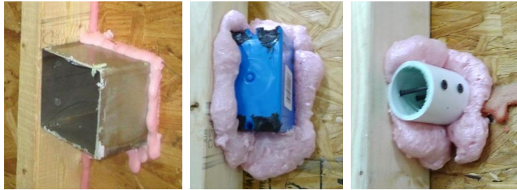
Figure 22. Penetrations through OSB sealed with latex foam sealant or canned foam.
