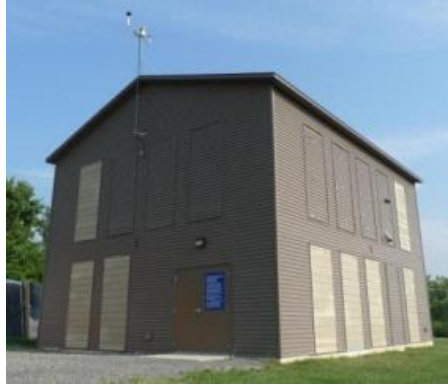
Figure 2. Building Envelope Systems Testing (BEST) lab.
