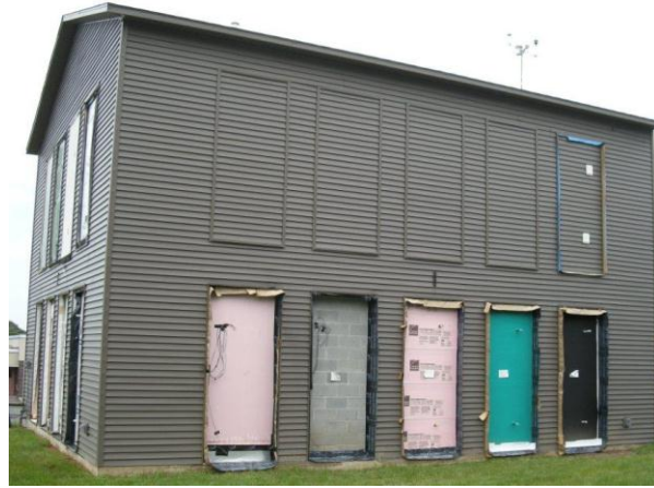
Figure 1. Building Envelope Systems Testing (BEST) lab.
