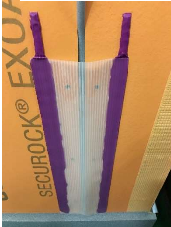
j. Bridging a joint in a wall
