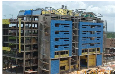
o. Completed air barrier project
