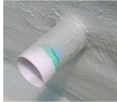
h. Properly detailed round penetration
