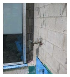
When designing the connections between different building assemblies and to different air barrier components, keep in mind that the movement of these materials when subjected to temperature changes and moisture content changes. As the two different materials will move at different rates, this has to be accommodated. An example would be an aluminum framed window set into a CMU back-up wall. The movement between the different materials will be severe.
